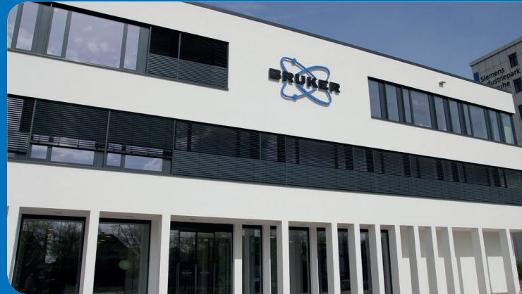
Bruker facility in Karlsruhe
